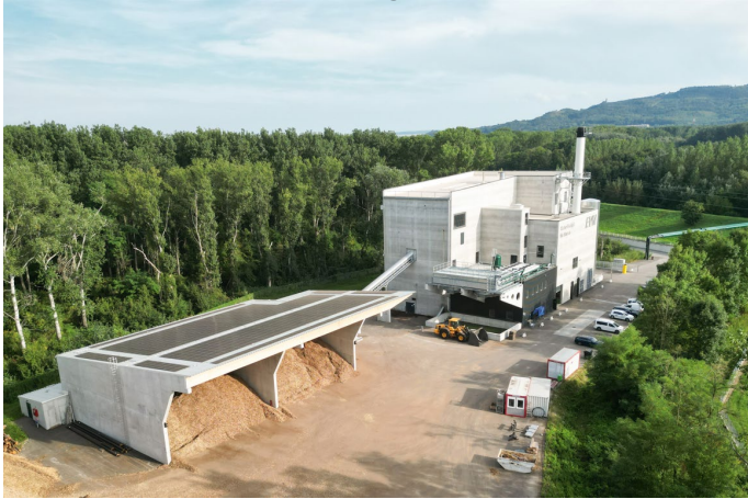
Biomass-fired cogeneration plant
