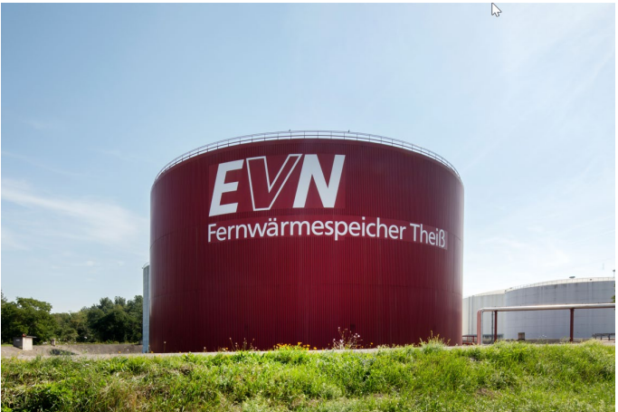
Hot water storage
